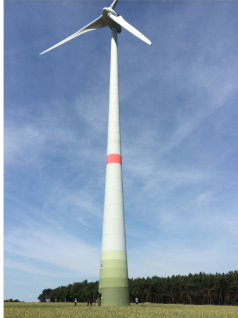
Figure 2. CREATE Participants enter the base of an Enercon turbine at the Feldheim wind farm.
