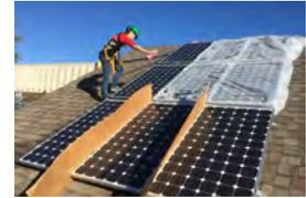
Panels were spray coated in the field rather than removing and replacing them. UV rays from the sun dry the solution and sinter the silica and titania to crystallize their structures and chemically bond the coating to the glass.
